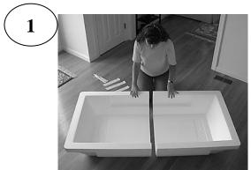
1) Lay Draft Cap upside down on flat, protected area. Align halves end to end, and align sides.
