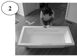
2) Apply tape to the flat surface as shown.
